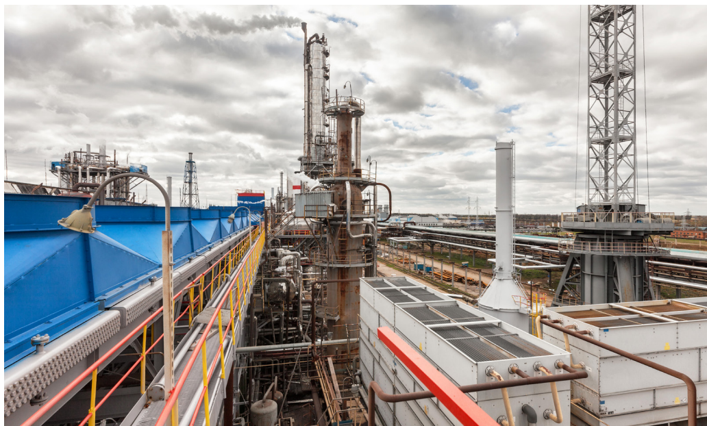
Industrial plant that makes ammonia
