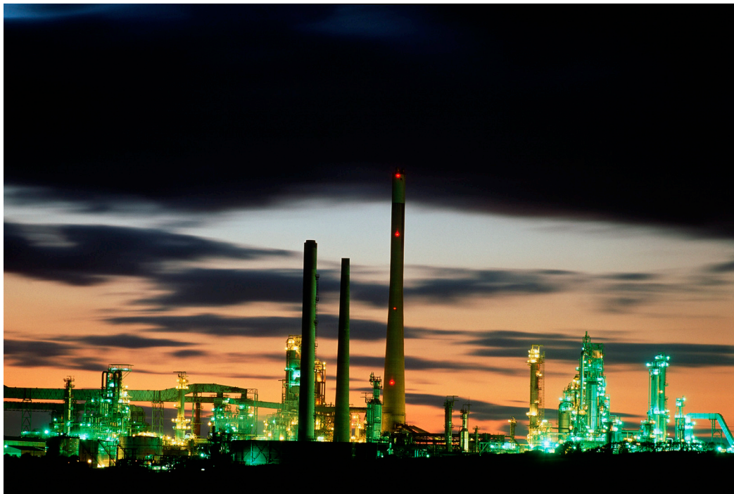
Oil refiner , Milford Haven Martin Bond / Science Phoyo Library
